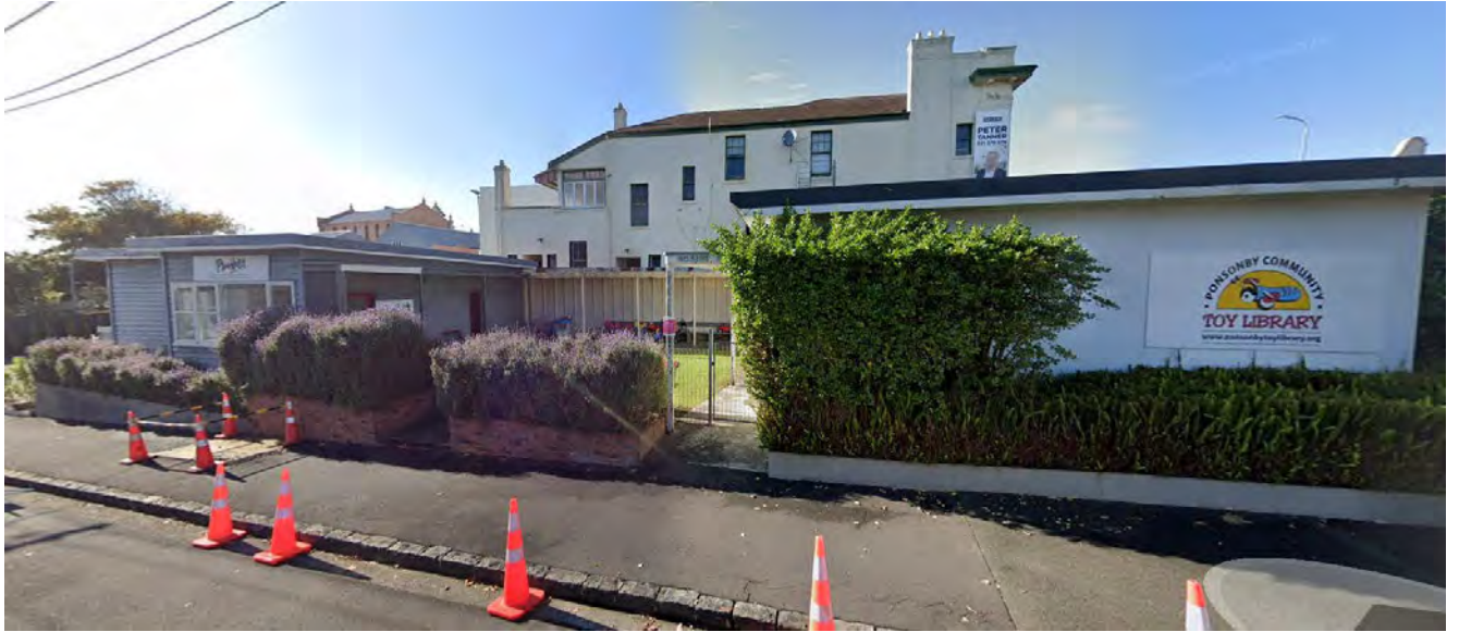
Figure 2: Street view of 19 Jervois Road from Deadwood Terrace
