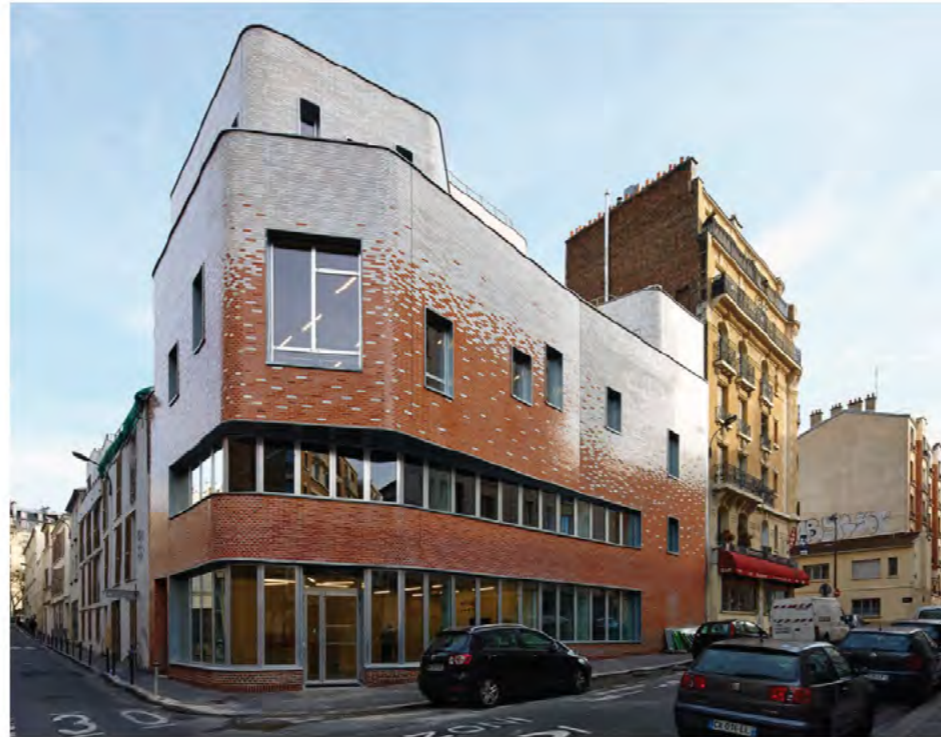
The Victor Gelez Community Centre / Dumont Legrand Architects https://www.archdaily.com/508386/the-victor-gelez-community-centre-dumont-legrand-architects?ad_medium=gallery
