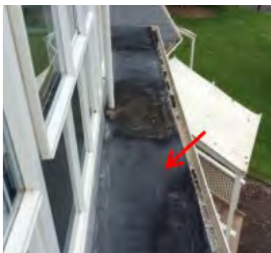
(Asbestos Containing Bituminous Membrane Example)
