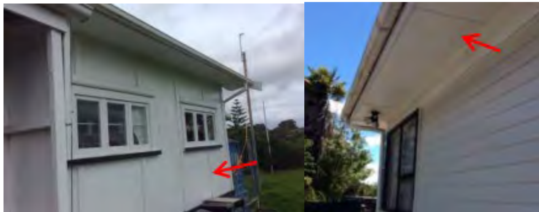
(Asbestos Containing Cement Sheet/Cladding and Soffit Examples)
