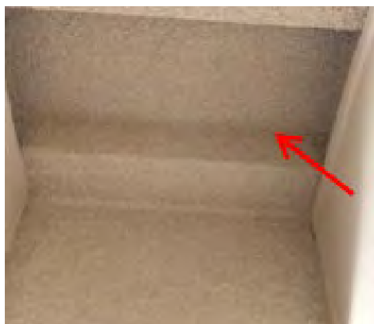
(Asbestos Containing Sprayed Material Example)
