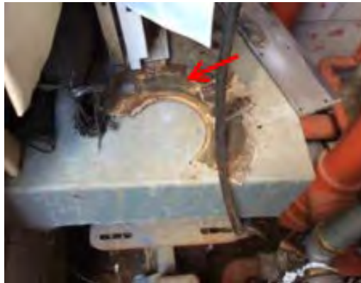
(Asbestos Containing Gasket Example)
