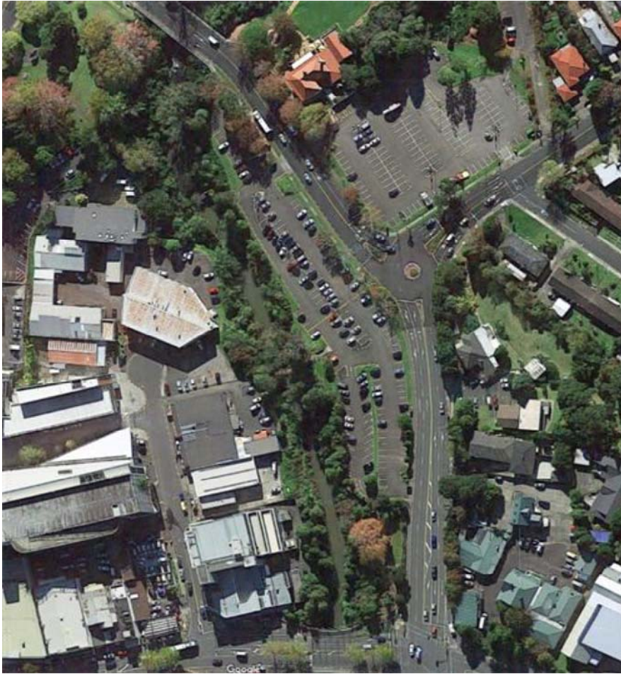
Figure 3. Aerial view of the Falls & Alderman Carparks, showing proximity to the Wai Horotiu Stream
